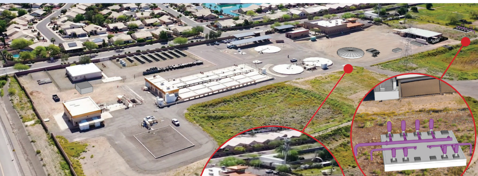
Beardsley Water Reclamation Facility
